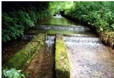
Photo 2. Diversion work A
