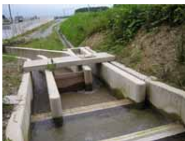
Photo 3. Diversion work B
