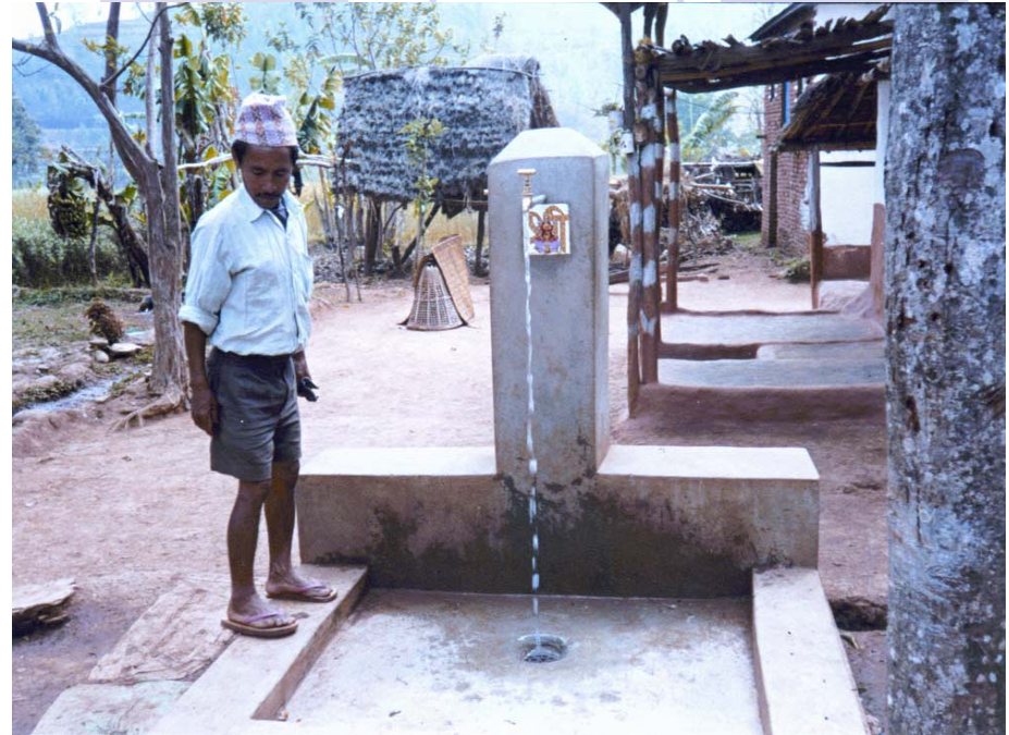
Maintenance Worker repairing the Tap Post
