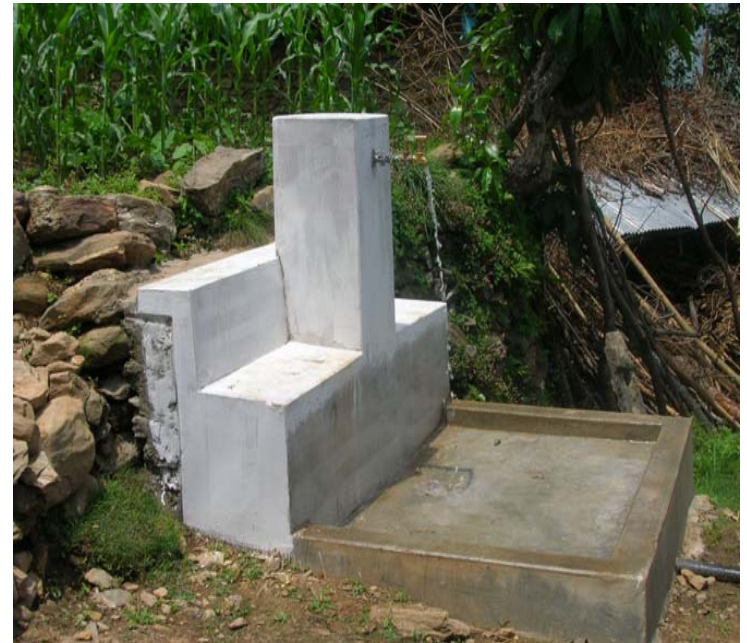
Water Supply Tap Post
