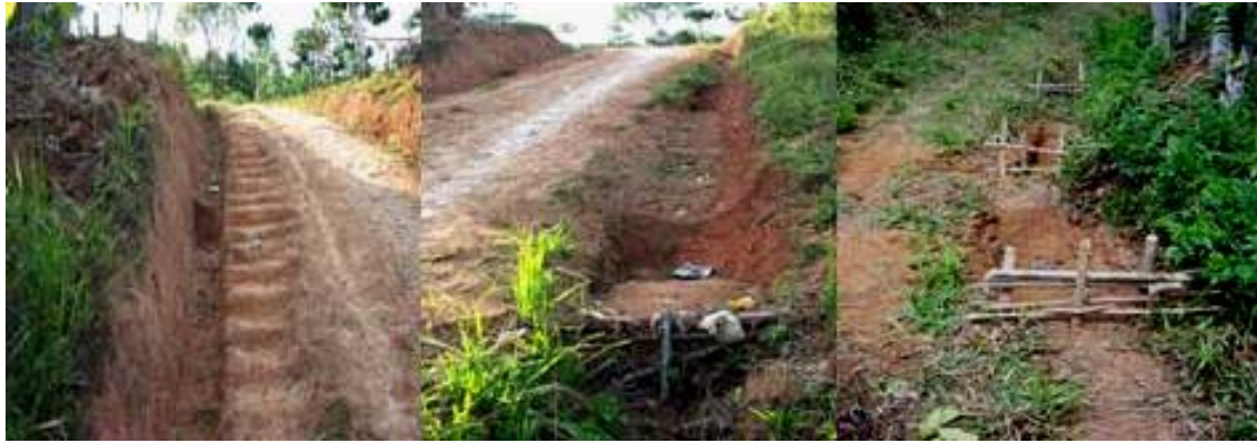
Figure 2. Simple structures to reduce runoff and trap sediment on public footpaths
