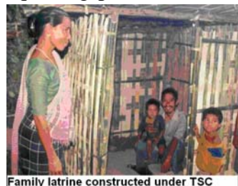
Family latrine constructed under TSC
