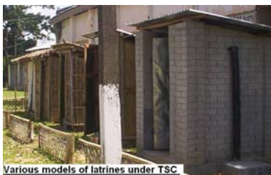
Various models of latrines under TSC
